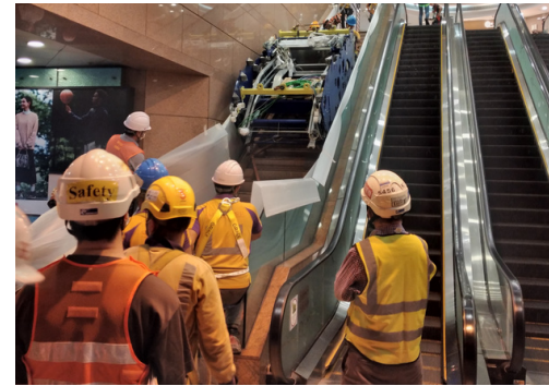
Introducing escalator head pieces in C.C. Telford Garden (Hong Kong)
