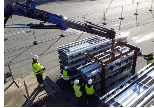
Moving walkway works (unloading) - Oslo Airport (Norway)
