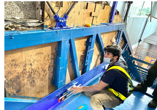
Precision level works on structure supports in Johor Bahru (Malaysia)
